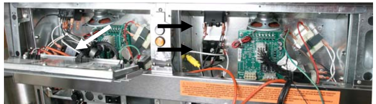
FIG. 1: A transformer in the left box (see left arrow) is replaced; new relays are shown in place (see arrows). A plastic bushing is placed in an existing hole below the time-delay relay in the control box.
