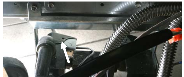
FIG 2: The fill RTI solenoid (left as viewed from back) is wired to the relay system installed in the control boxes.
